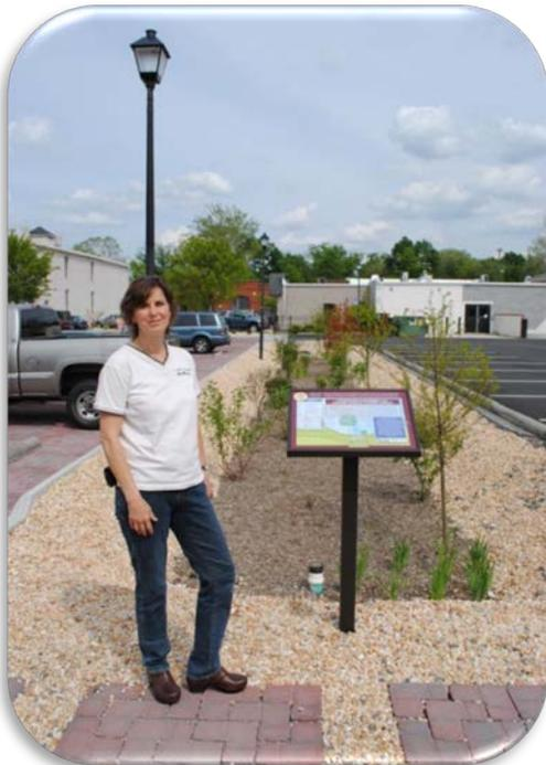
lot. The newly reconstructed lot is one of the first to combine permeable pavers with rainwater storage beneath and a commercially-produced bioretention device in the parking island to slow down, capture, and treat polluted rainwater and snow melt. It provides enough capacity to fully store and treat all of the rainwater from a typical 1-inch storm event—along with a usable parking lot and improved curb appeal.
